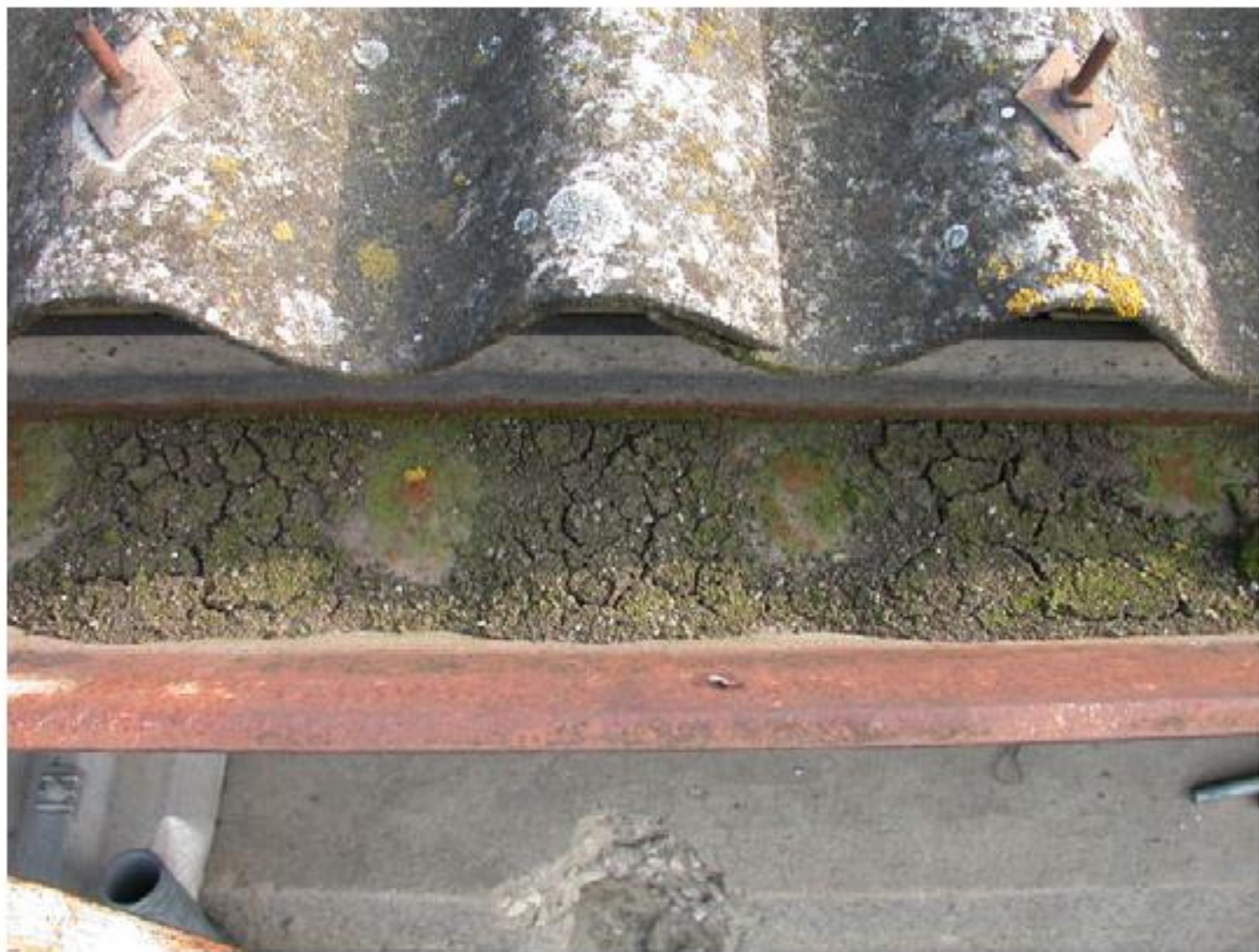
Fig. 2. Friable material in the gutter.
